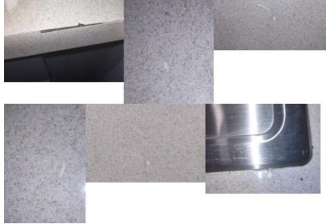
Scratches for installation of accessories.
